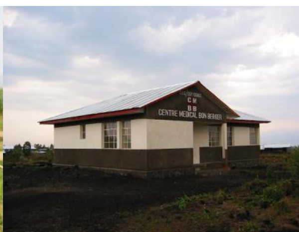
S4: SANRU III began with a relief phase funded by OFDA. Some of these funds were used to construct and equip the Bon Berger Health Center (above) near Lake Kivu, Goma where an existing structure had been destroyed by a Volcanic eruption.
