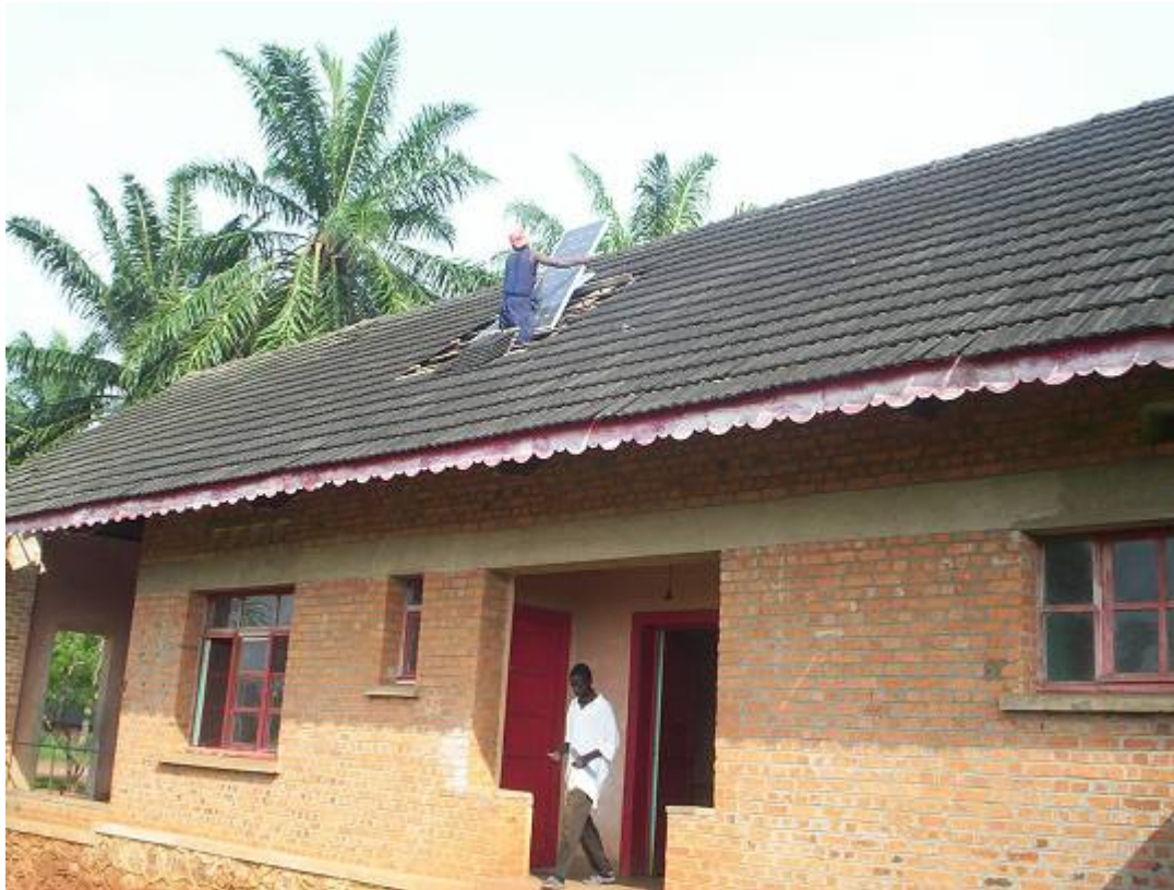
Picture 6. Renovated Health Center, Karawa Health Zone
